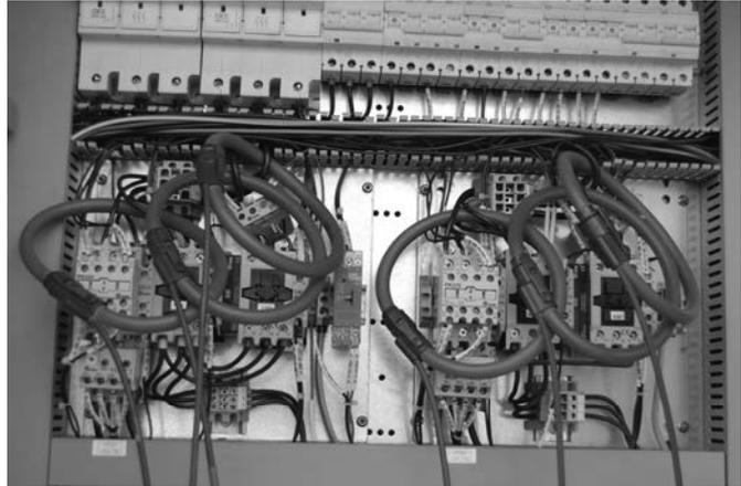
**Fig. 7** Current loops of The ENA 500.22 analyser
