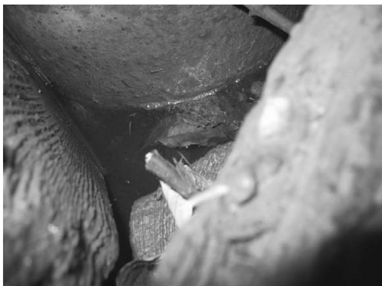
Fig. 4. Research Position No. 3. The well has wooden casing preserved; see the section of pipe casing; the commune of Iwonicz-Zdrój, Subcarpathian voivodeship, 2011 (photo by Lipińska E. J.)
